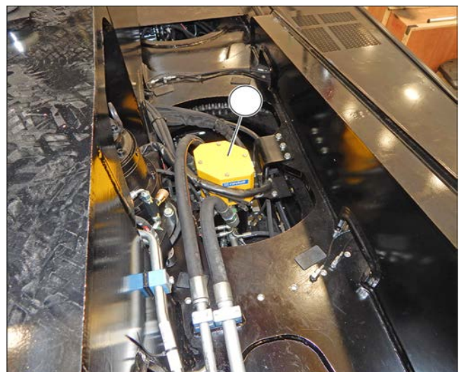
Figure 224: Check and cleaning of the transmitter rings of the rotating electric collector
